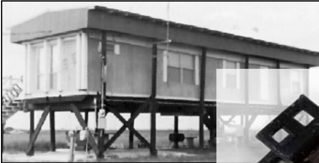
Manufactured Home Showing Cross Bracing and Foundation.
