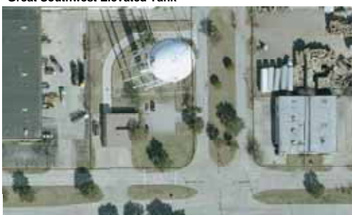
Great Southwest Elevated Tank
