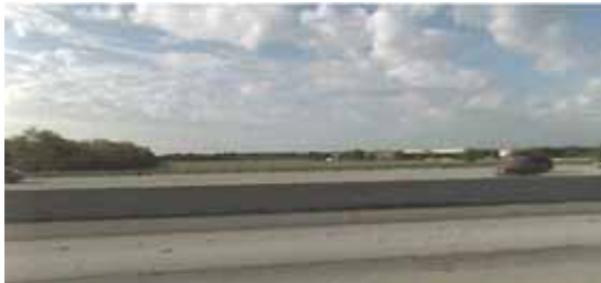
Center Street Bridge @ IH20
