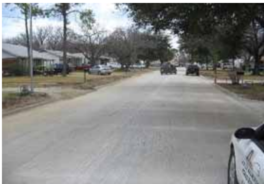
Residential Street Rebuild
