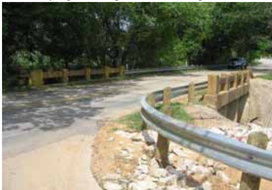
Bowman Springs Rd Realignment & New Bridge
