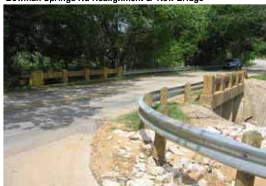
Bowman Springs Rd Realignment & New Bridge
