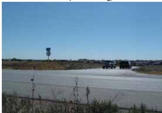
Collins St. at Debbie Lane (Harris Crossing)
