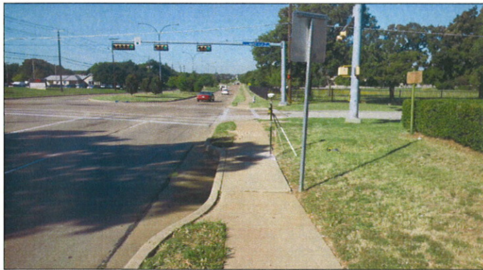
FACING WEST TOWARDS MONUMENT
